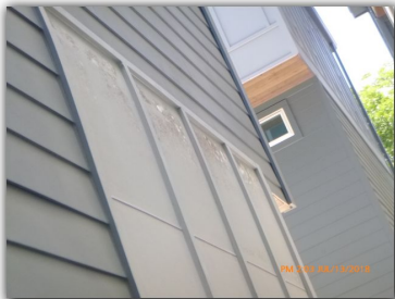
Unfinished areas that are not painted, front edge, behind condenser.
