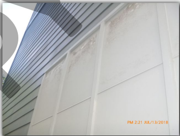
Unfinished areas that are not painted, front edge, behind condenser.
