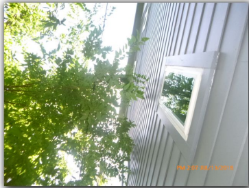
Foliage should be trimmed back away from exterior walls.
