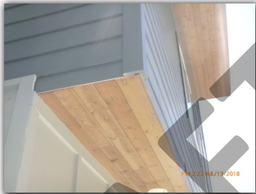
Siding has lifted out.
