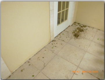
Stucco into grade and into patio slab, no weep screed.
