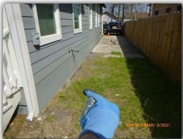
Splash-blocks missing at several down-spouts.
