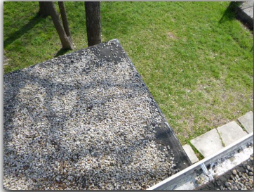
There are areas with exposed tar (tar is dry and cracked) unprotected tar is susceptible to the elements, repairs are anticipated.
