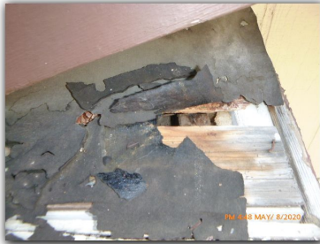
Damaged / missing shingles:
