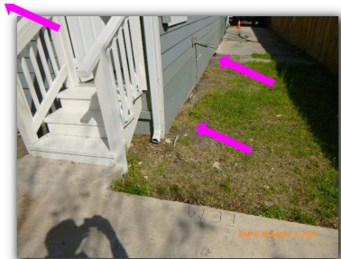
Splash-blocks missing at several down-spouts.
