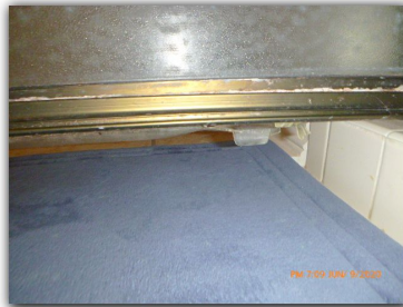
Door sweep is damaged.
