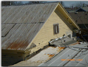
Tin roof is rusted, loose and patched with different type of roofing material and very old.
