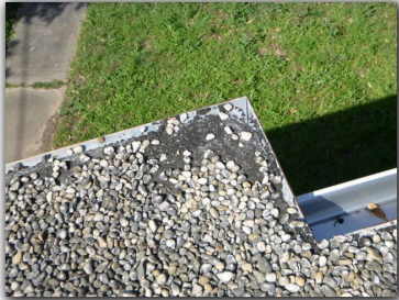
There are areas with exposed tar (tar is dry and cracked) unprotected tar is susceptible to the elements, repairs are anticipated.
