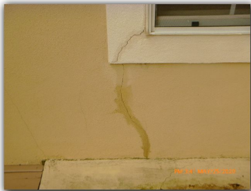
Silicone caulked cracks.
