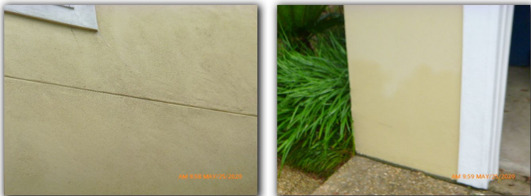
Cracks and moisture intrusion:
