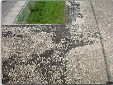
There are areas with exposed tar (tar is dry and cracked) unprotected tar is susceptible to the elements, repairs are anticipated.
