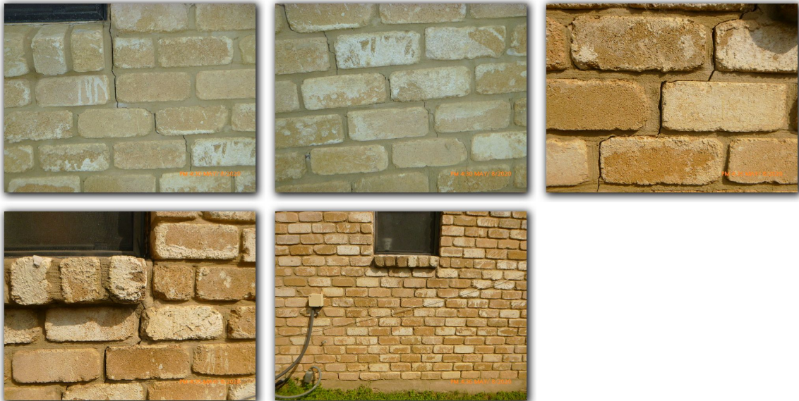
Cracks in brick;
