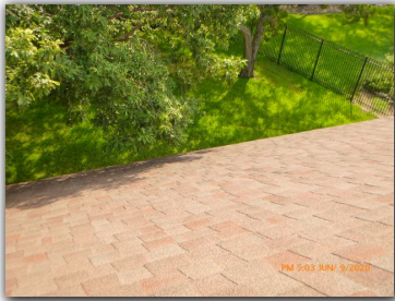
Tree limbs and branches should be cut back 3' from roof line.
