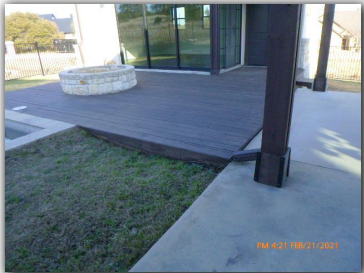
Potential for water to pond at deck between patio and pool.
