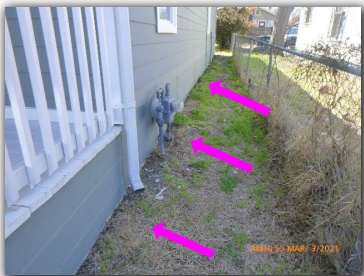
Splash-blocks missing at several down-spouts.
